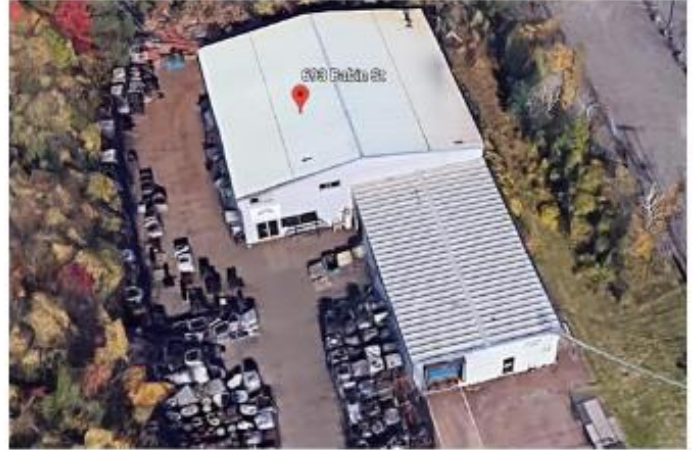
Factory, Dieppe, NB Canada
